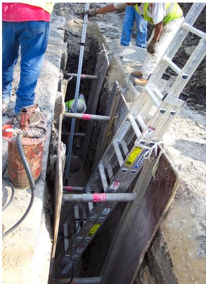
**Figure 1.** Work crew installing water pipes. Aluminum hydraulic shoring is being used as a protective system for the trench. *Photo courtesy of George Kennedy, NUCA.*
