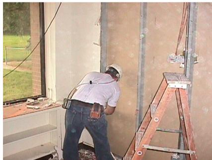
Operation such as cutting, sanding and drilling of products containing man-made mineral fibers can also produce dust. Control through the use of tools with dust capture systems and hoods incorporated into the tools are often the best solution. Spraying surfaces with water reduces fiber generation. Housekeeping practices such as use of HEPA vacuums instead of dry sweeping can also reduce potential exposure.
