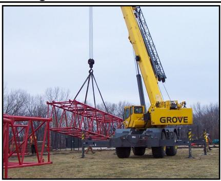
The photo above shows a crew assembling a lattice boom crane using a hydraulic crane to lift the boom sections. Every year many workers are injured or killed working around cranes. To help reduce accidents, crane operators should be certified and riggers and signal persons should be qualified for the tasks they are performing. Review this photo with your crew and discuss the hazards noted. In the section below list the hazards and the controls that may help reduce or eliminate them.
